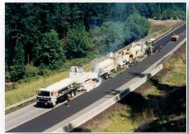
Cold Recycling (CR) is a asphalt pavement rehabilitation technique that typically consists of rehabilitating 2-6 inches of the existing pavement. CR Options include:
