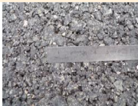
Surface E1: Semi-granular bituminous concrete (0/10)
