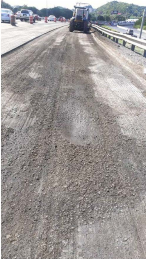
Suspect area after milling
