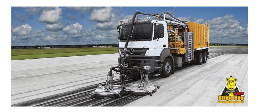
Shotblasting: Process that uses an abrasive material to blast rubber off runway pavement surface.
