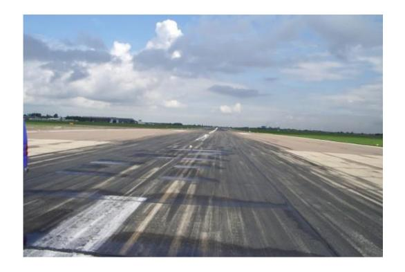
Chemical Removal: Chemical compound to soften and decompose the rubber so it can be gently removed by a broom or vacuum.
