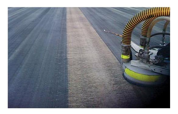
Mechanical Removal: Scraping, grinding, milling or sandblasting to remove rubber buildup.
