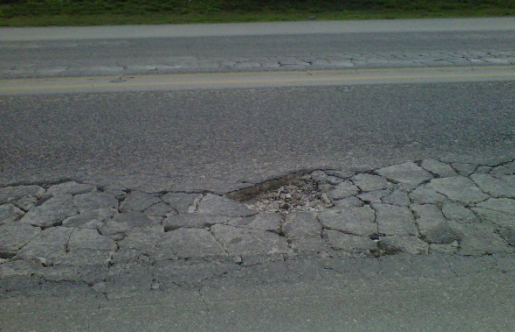
Base Failures
