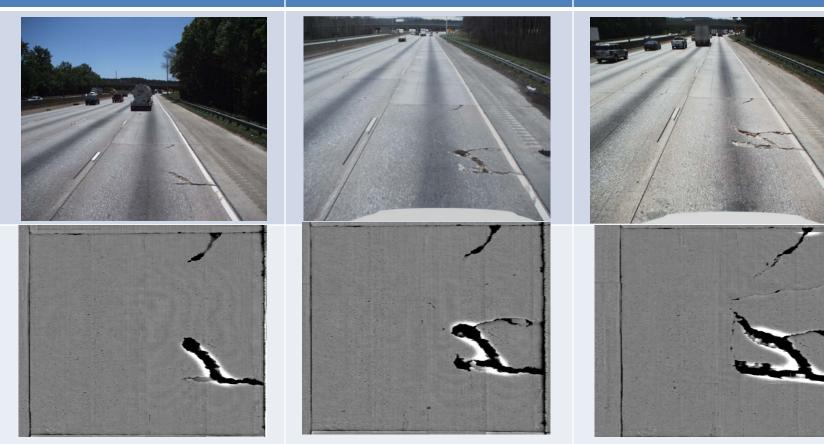
Transverse Crack Level 2Length:7.4 ftMax. Width:138 mmMax. Depth:47 mm
