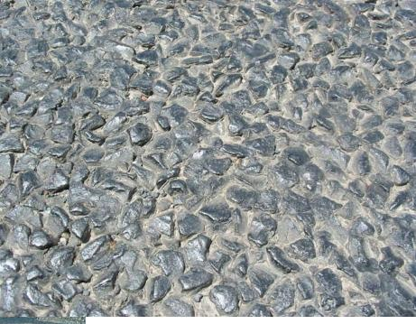
95% of all sealed roads in New Zealand are chipseal over unbound granular pavements
